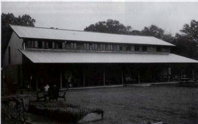
Straw bales were used to build the 5,000-square-foot house, with the students assisting. One can grow three such houses in 1 year, as opposed to a wood-frame house, which takes about 30.
